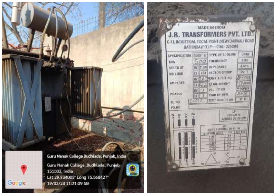
Main LT Distribution Transformer
